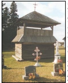
Plate 26. Bell tower of St. Alias church, Sirko. The roof of the tower is built of roughly laid vertical shakes similar in nature to planking. Bell towers were a ubiquitous feature on Ukrainian churchyard in Manitoba, just as they had been in Ukraine. Those in Manitoba were, like this one, simply constructed and animated with a few functional, but decorative elements.
